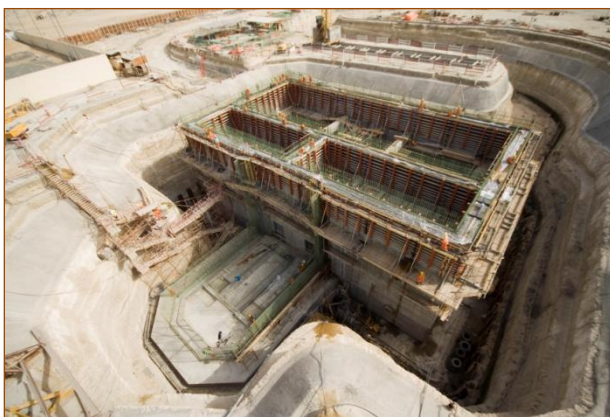
Pumping Station Works (Dubai)
