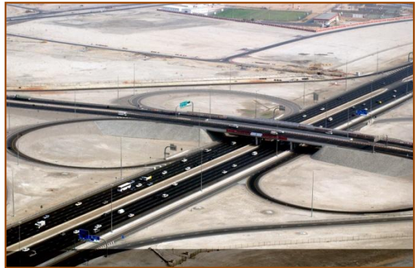
Mamzar Interchange (Dubai)
