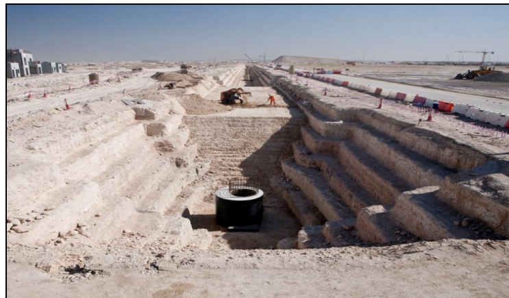
Deep Excavation Works (Al Falah, Abu Dhabi)
