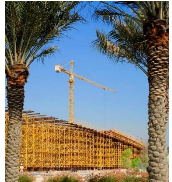
Wade Adams Contracting LLC, Dubai Improvements of Al Safooh Roads
