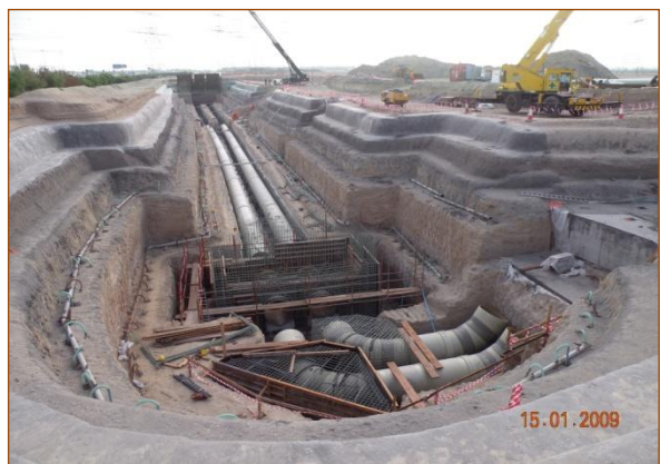
Pumping Station Works (Dubai)
