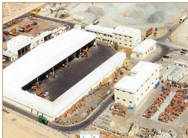
Wade Adams Workshop and office facility (Dubai)
