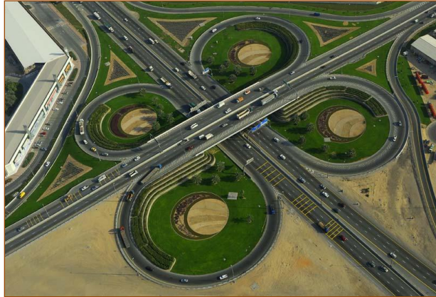
Ras Al Khor Interchange (Dubai)
