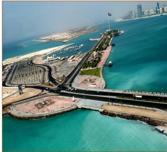
Break water developments (Abu-Dhabi)
