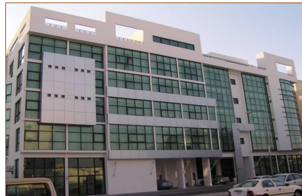
Residential Building at Umm Al Hassan (Bahrain)
