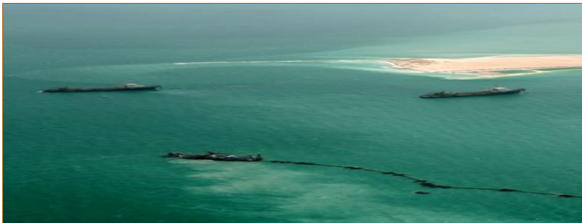
Land reclamation (Bahrain)
