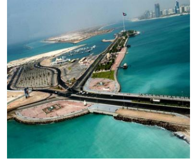
Hilalco, Abu Dhabi Breakwater developments Project
